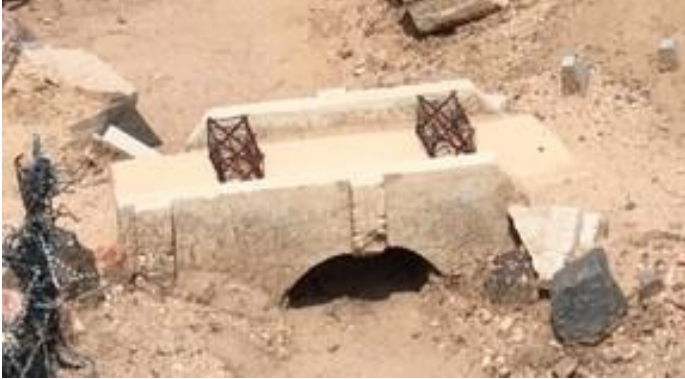
Bridge Barricades (soldered brass strips w/ wire wrapped around).
